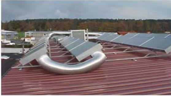
**Fig.1.** passive solar air chimney
