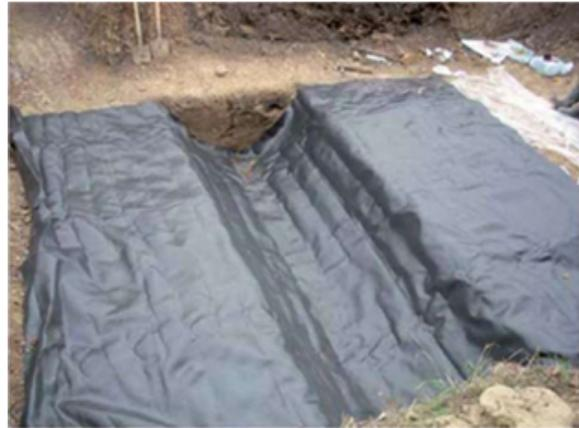
Fig. 1: Reinforcing material installation process.
